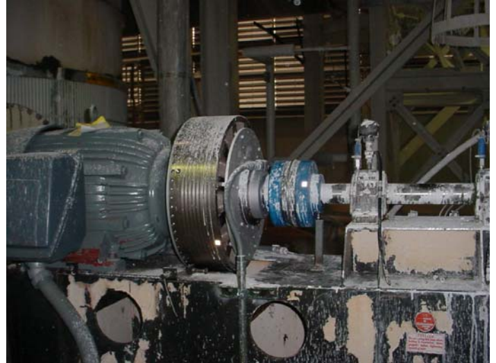
125hp "Pro" PAYBACK® direct coupled VSD Soda Ash Plant, Colorado
