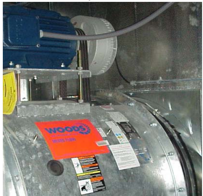
40 HP "Easy" PAYBACK® Variable Speed Belt Drive for Woods Fan, factory installed, Dallas, Texas
