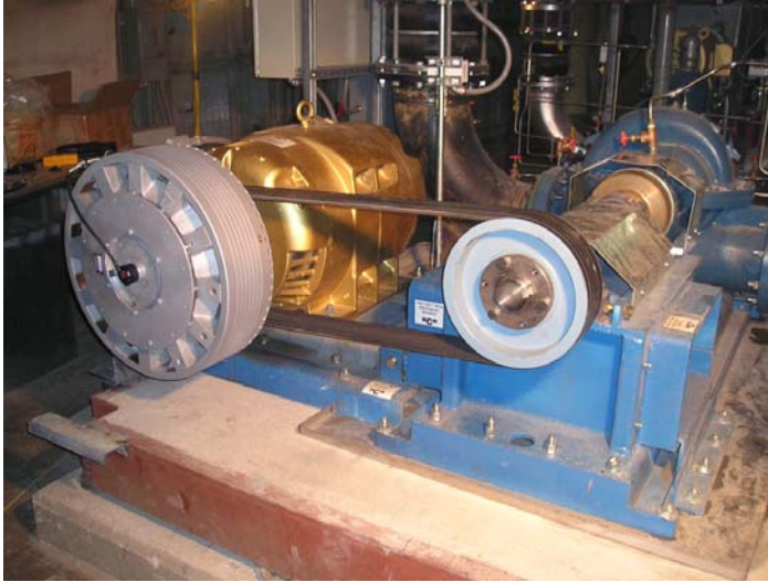
150 HP Easy PAYBACK®VSD chilled water pump. Houston International Airport
